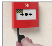
Step 3: To reset a simple key is inserted into the bottom of the call point.
