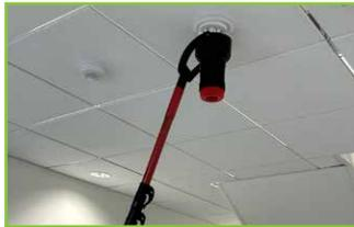
6. Place the head over alarm and begin testing by pushing upwards for one second.
